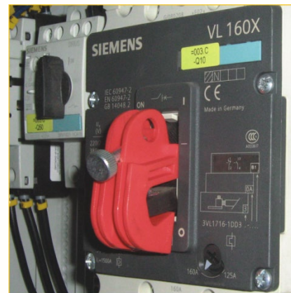
CB-UNI-HT (MCB & MCCB Lockout)
