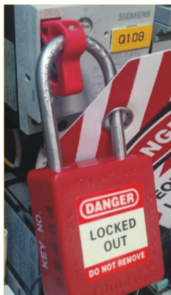
UB-CTBL (MCB Lockout)
