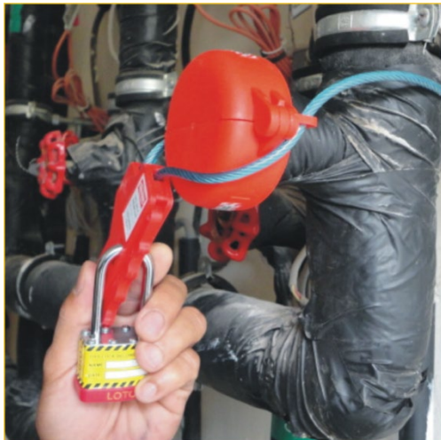
SMCL+1M Cable Lockout (Gate Valve)
