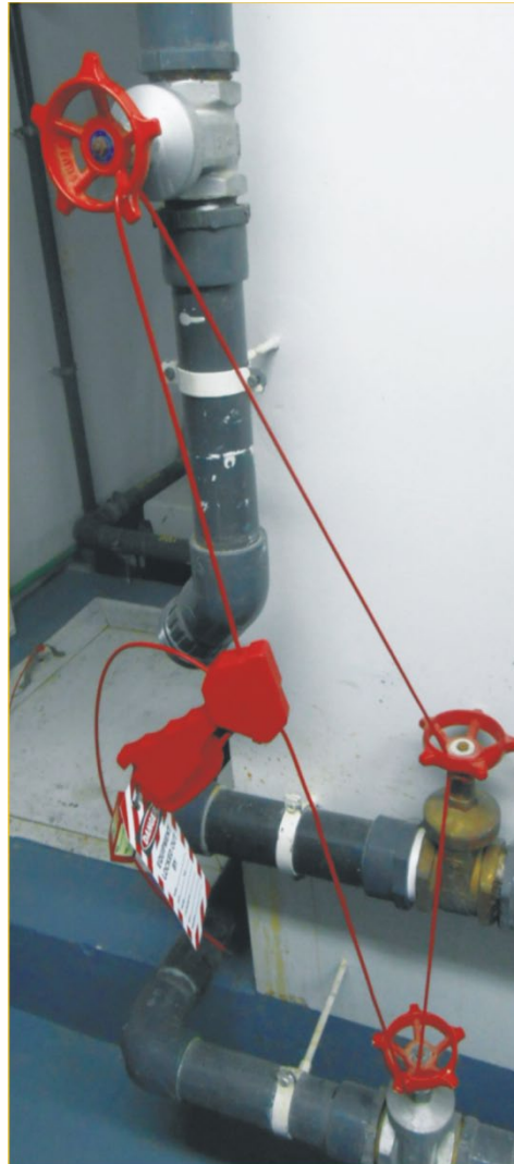
CL-PSM-2M Cable Lockout (Gate Valves)
