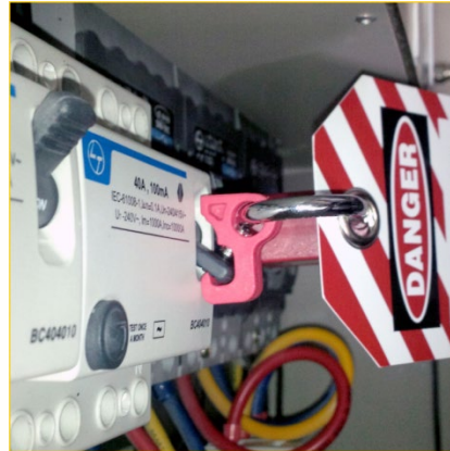
UB-CTBL (MCB Lockout )
